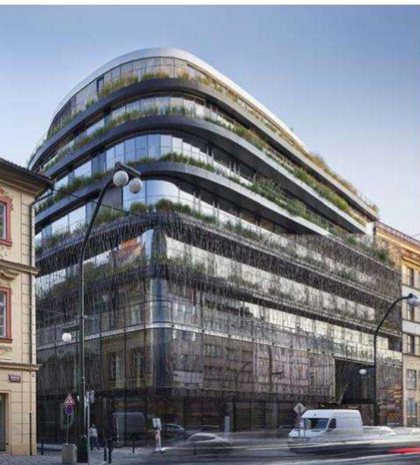
"DRN" in Prague, one of our most recent acquisitions
