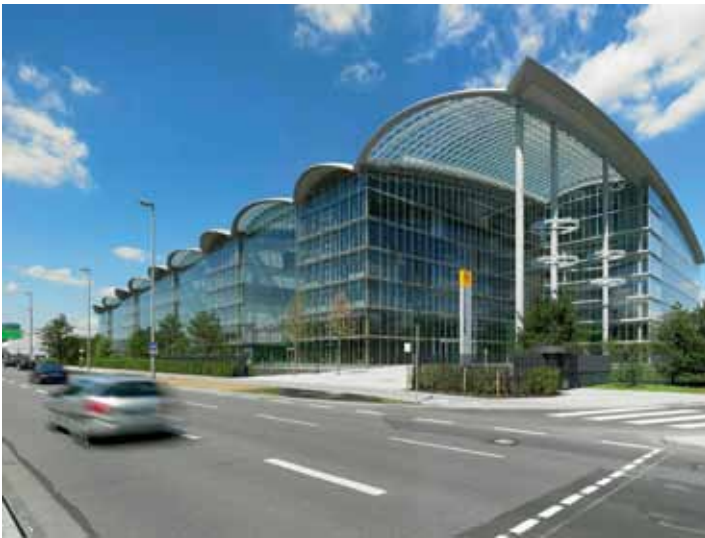
Lufthansa Aviation Center, Büro; Frankfurt/M.
